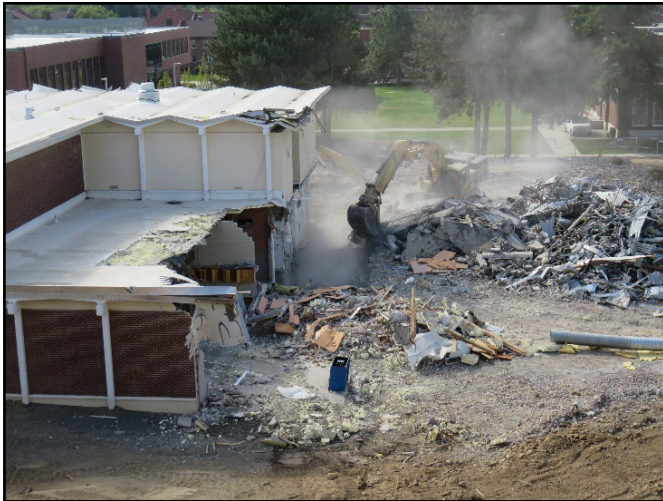
Hertz Hall demolition
